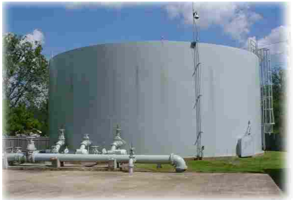
Ground Storage Tank
