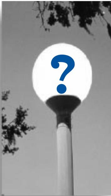
After the drinking water is treated, the pure, germ-free water is pumped through pipes to customers. The water tower is attached to these pipes under pressure so that the extra water simply goes up the pipe into the storage tank automatically, and comes back down when it is needed. At night, when the demand for water falls to practically nothing, a pump can help to refill the water tower to be ready for early morning demand again. ♦
